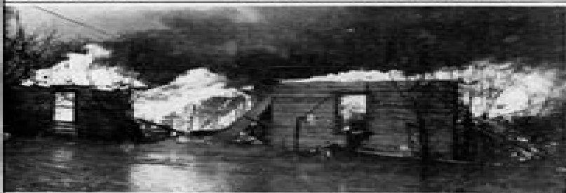
Tuesday blaze A Bastrop woman with eight children was left homeless when an early morning fire spread through the second-story structure. Firefighting units were located within 100 feet of the burning structure. The fire, which started in the second story of the home, spread to the first floor and the roof. The fire was extinguished by the Bastrop Fire Department. The woman and her children were rescued and are now in a local hospital. The home was destroyed.
