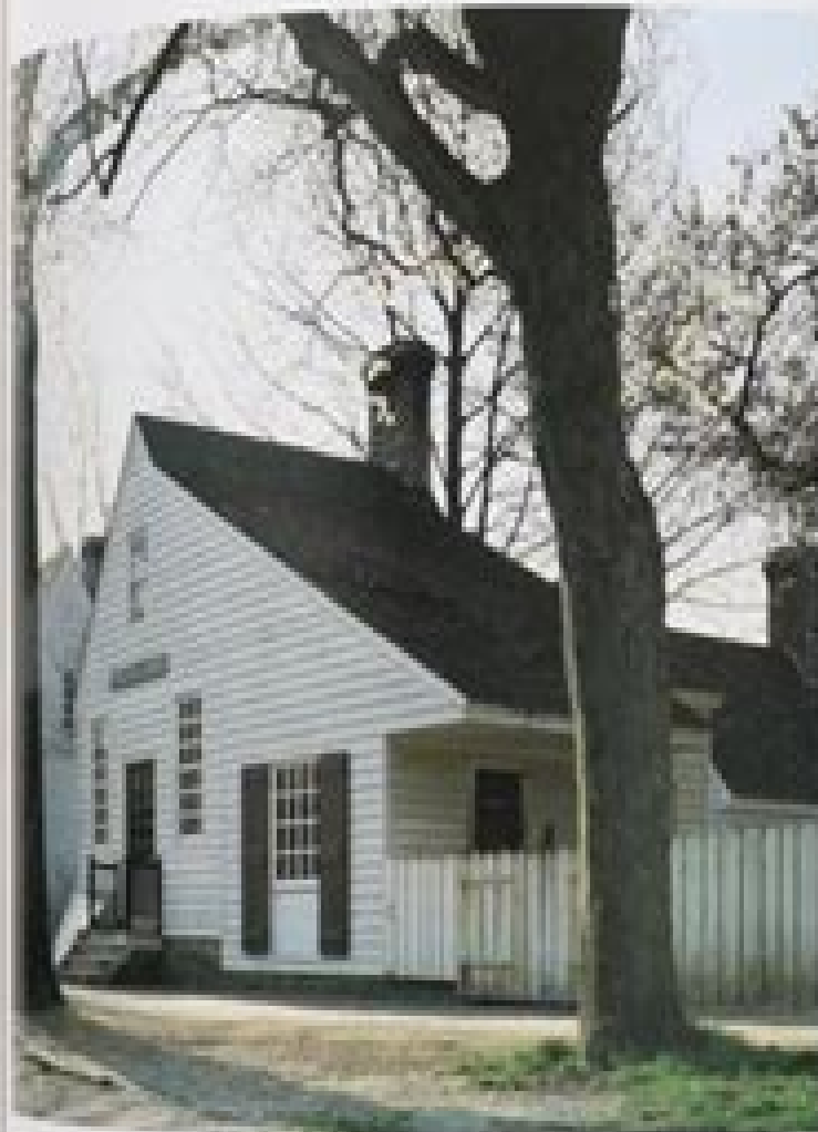
In 1981, the removal of the false front returned the facade to its original appearance.
