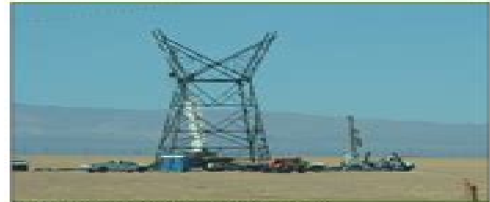
Transmission line tower construction site.
