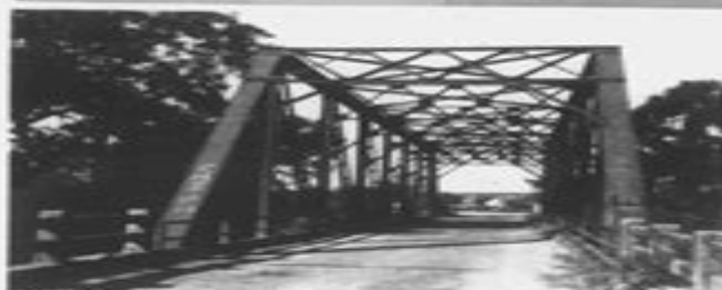
THIS OLD IRON BRIDGE on the airport road, is scheduled for replacement next year in a Texas Highway Department project, with the City of Coleman as local sponsor. The old bridge, spanning Hards Creek, is commonly known as the old Burkett bridge, so the route was formerly the Burkett Highway.
