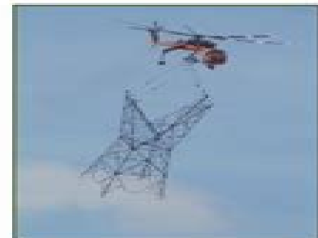
A sky crane helicopter carrying the top section of a LST.
