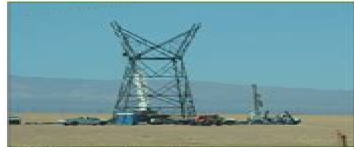
Transmission line tower construction site.
