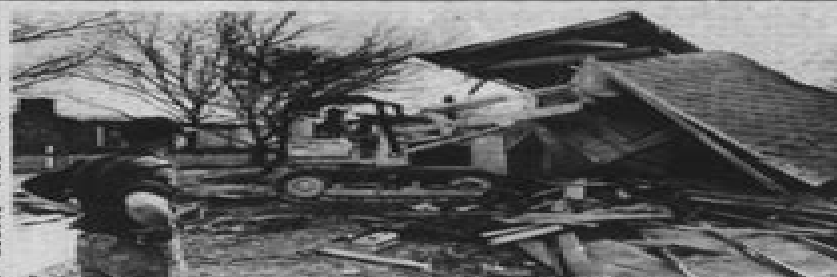
REPAIRS TO North Brownwood Baptist Church, destroyed by fire, are being made by the North Brownwood Baptist Church. The church is being repaired by the North Brownwood Baptist Church.
