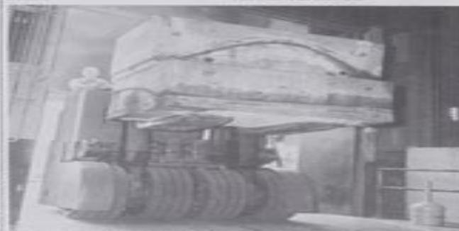
MONSTER—Newest addition to Convair Fort Worth's rolling stock is this 40,000-pound capacity lift truck. Here S. E. Allen of traffic men truck loaded with metal die on truck enters south end of plant. One of only three such in U. S., truck may be driven from either side with dual control. Largest lift truck at Convair SD has 20,000-pound capacity.
