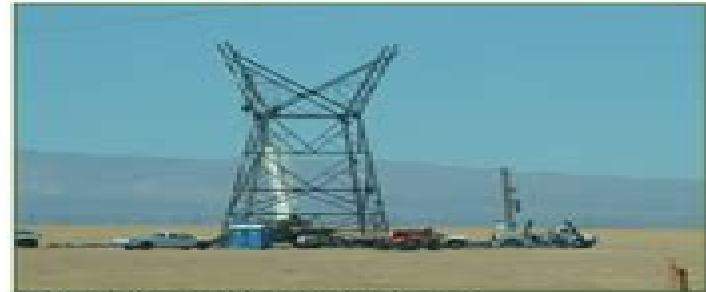
Transmission line tower construction site.
