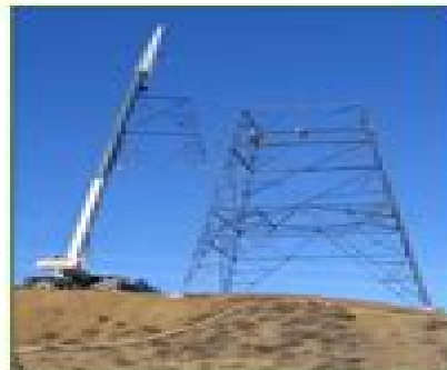
A crane carrying the top section of a LST for installation.
