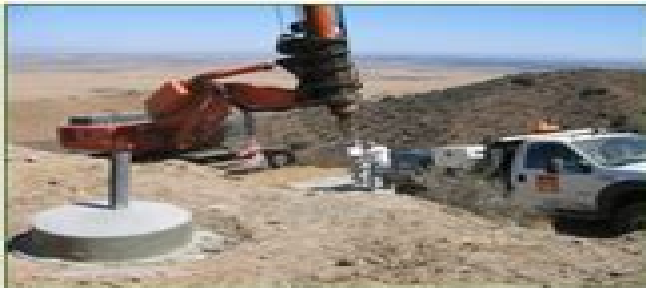
Foundation construction for an LST.
